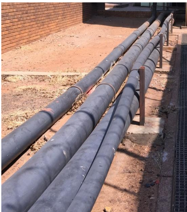
Figure 2-4: Steel Pipe Supports
